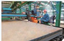
200厚钢板切割 200 thick steel plate cutting
